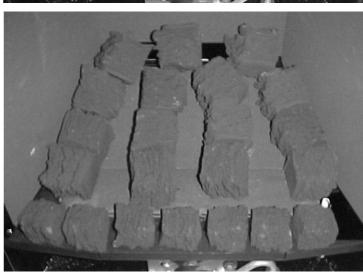
Add 5 55mm x 55mm coals on the front row resting between the 35mm coals and 45mm coals already placed. as shown. Place the end 2 square to the firebox sides and place the middle 3 at an angle. Place the coals with rough sides upwards. DO NOT allow the coals to fall through onto the burner or base board, they must be placed on top of the coals already fitted.
